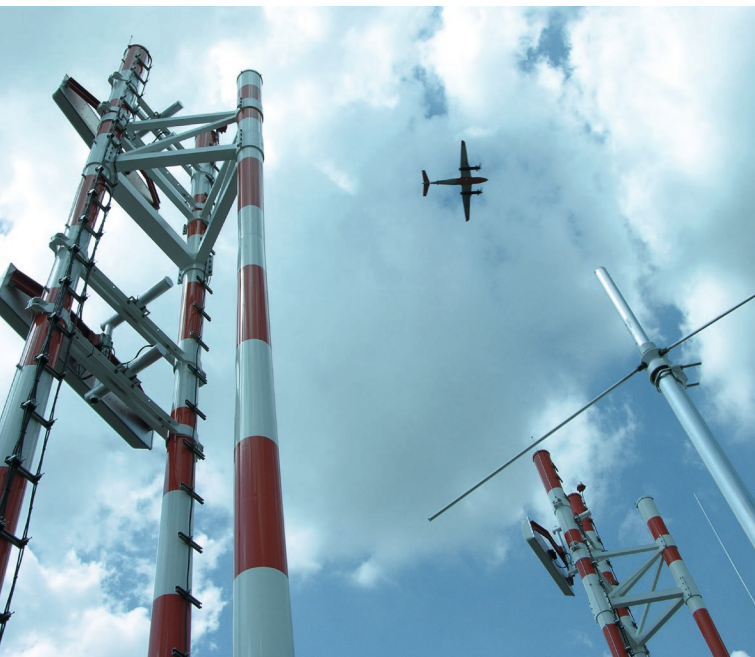
Glide Slope Transmitter Frankfurt Airport, Runway Northwest (Photo: FCS)
